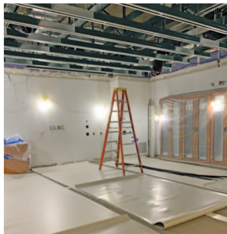
Cath Lab renovations underway
